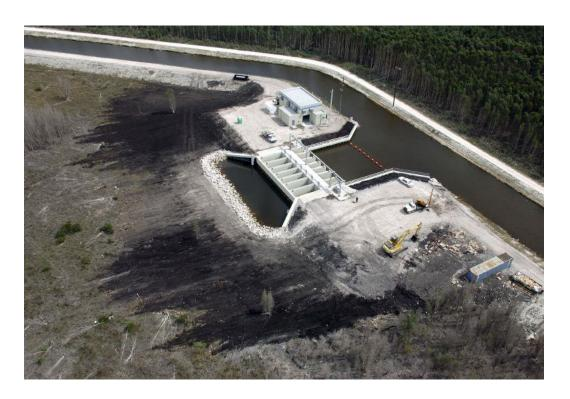
The EDB is two reservoirs of nearly 500 acres each Allows for storage of up to 4,000 acre/feet of water
