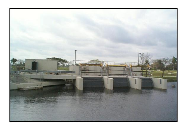
This pump is designed to push water against the tide
