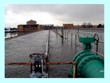
Treatment tanks overflowed at the Hunts Point (Bronx) WPCP during a March 2001 storm; unusually high tide elevations prevented discharge of treated sewage into the East River and caused back-up
