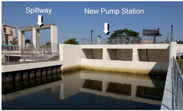
Forward Pump at S-26 Structure. Image Source: SFMWD
