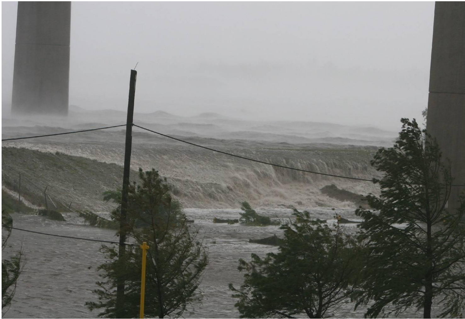
Picture taken by an automatic camera located at an electrical generating facility on the Gulf Intracoastal Waterway (GIWW) where the Route I-510 bridge crosses the GIWW. This is close to where the Mississippi River Gulf Outlet (MRGO) enters the GIWW. The shot clearly shows the storm surge, estimated to be 18-20 ft. in height..
