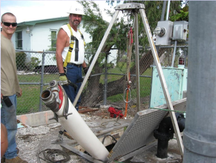
Gravity Sewer Lining
